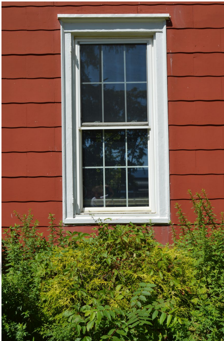
Photograph 6: Detail view of original window trim, looking northwest.
