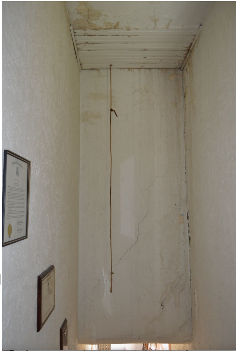
Photograph 12: Interior view of stairway from the second-story landing, looking east. Note the belfry trapdoor in the ceiling and the rope for the bellpull.
