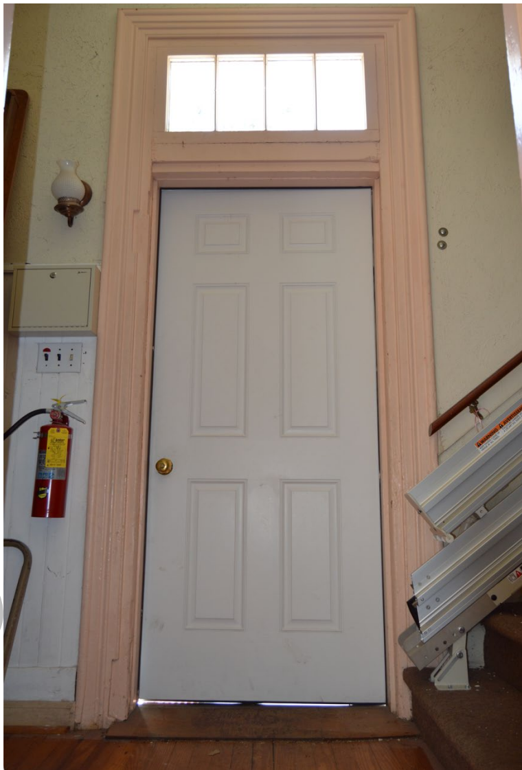
Photograph 8: Interior view of front door to vestibule, looking south.
