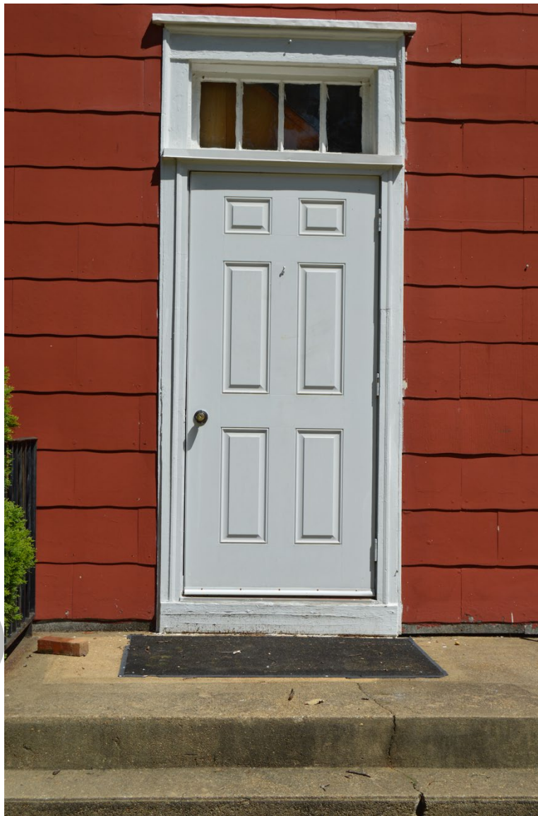
Photograph 5: Detail view of original transom above front door, looking north.
