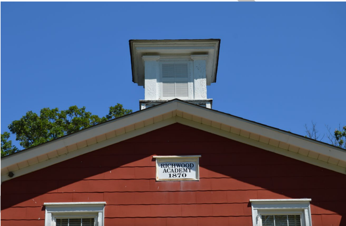
Photograph 4: Detail view of belfry and plaque on façade, looking north.
