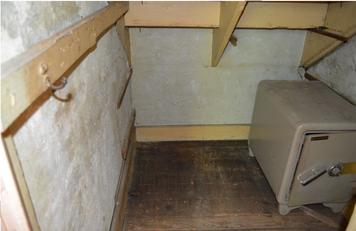
Photograph 11: Interior view of first-floor closet under the staircase, looking east. Note the original plaster walls and wood floors, which are covered over in the rest of the building, are visible here.
