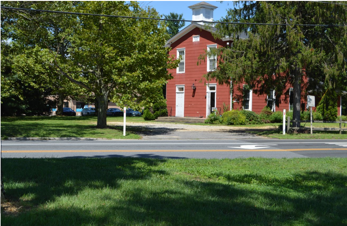
Photograph 1. Oblique view of Mount Pleasant School showing the façade and east elevation, looking northwest from Lambs Road.
