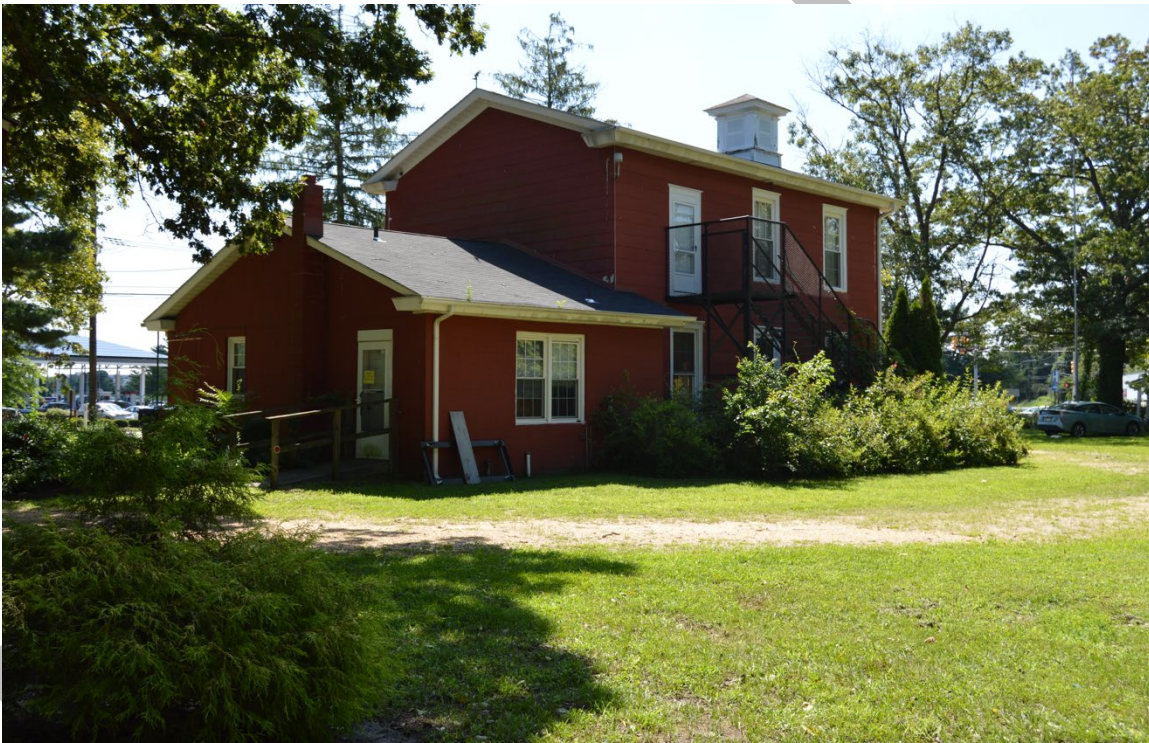
Photograph 3: Oblique view of Mount Pleasant School showing the north and west elevations, looking southeast.
